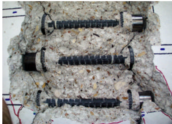
Figure 9-12: Internal cracking with hairpin confinement (specimen LS-08-04.04-12-10(N)-1-H0.6)
