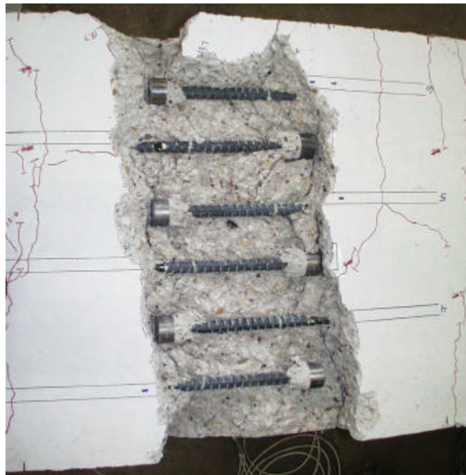
Figure 9-2: Photograph of failed lap splice specimen with cover removed from lap zone (specimen LS-08-04.04-12-10(N)-1)
