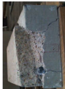
iv. Front View - Internal Cracking
