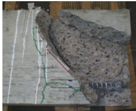
iii. Side View - Internal Cracking
